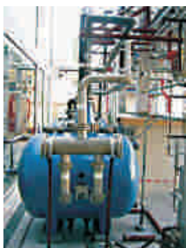
Hydraulic flame arrestor with Raschka Engineering holding an exclusive manufacturing license for China market
