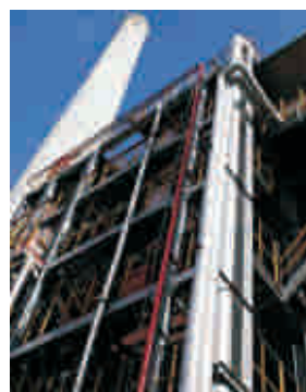
Incineration chamber with access platform, including steam generator with integrated steam blower to clean heat transfer area during operation
